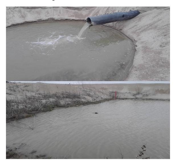
Flocculation occurred within 30 minutes or less, with clarity to the bottom of the pond.
